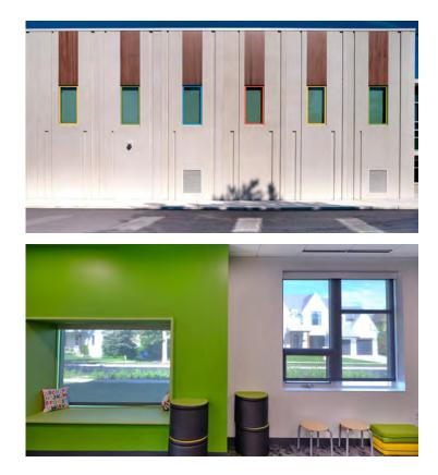
Winco offers a wide array of glazing choices and this project showcases that capability beautifully. Winco's clear anodized 3325 Zero Sightline windows are used in the curtainwall section of the building. The 3325 series is designed to allow occupants control of airflow and their overall environment.
